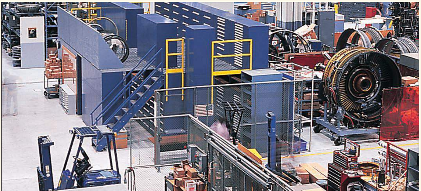
A mezzanine system can help increase throughput while freeing up floor space for other activities.
